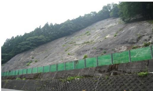
Figure.2 A large-scale slope covered shotcrete. (district A)
